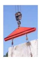
When working with slings, employers must ensure that they are visually inspected before use and during operation, especially if used under heavy stress
